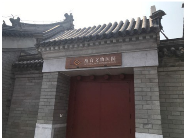
Hospital for Conservation, Palace Museum, Beijing.
